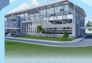
National Assembly Budget and Research Office (NABRO), National Assembly complex Abuja
