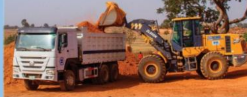
Construction of the 35km World Bank sponsored Access Road projects (RAAMP) in plateau state
